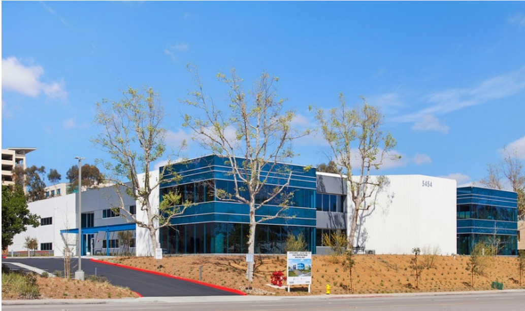
The renovated flex building at 5454 Ruffin Road in San Diego.
